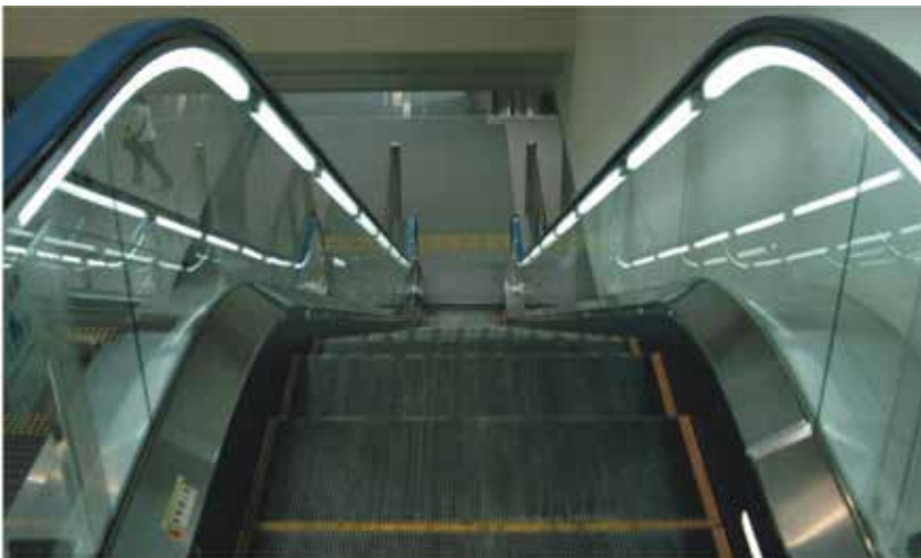
Handrail Lighting (optional)
