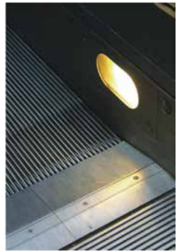
Comb Plate Step lighting
